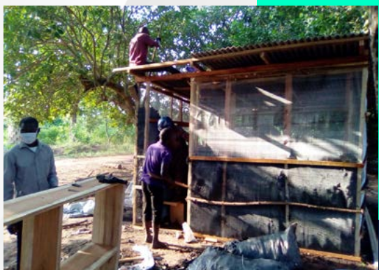
Construction of Charcoal Chiller at Ayete Zone in Ibarapa North LGA.
