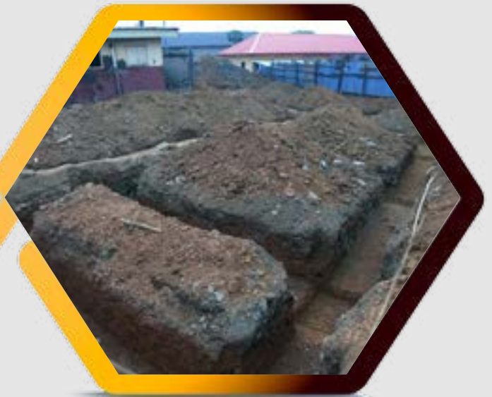
Reconstruction work of the PHCC at Idi Ogungun Ward 4
