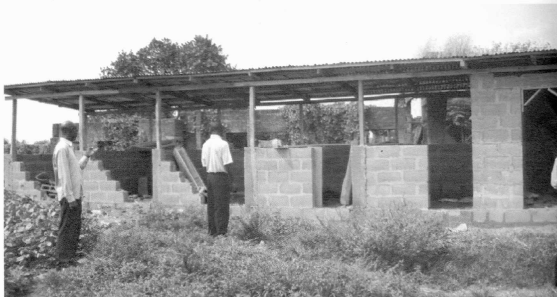
The UPA Pilot Project under construction at Ibadan North Local Government
